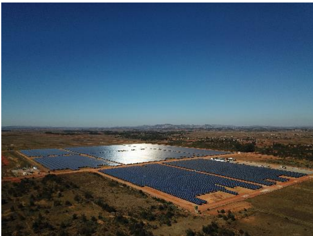
The largest Malagasy ground-mounted solar plant of Ambatolampy built by GreenYellow (20 MWP)
